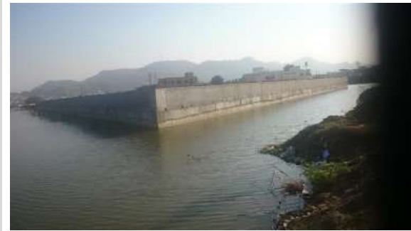
Submerged STP plant
