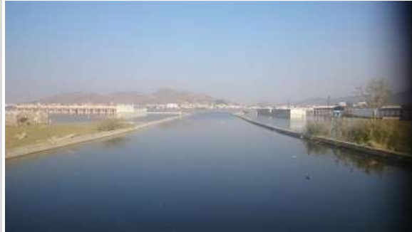
Inlet drain flowing from Foyasagar
